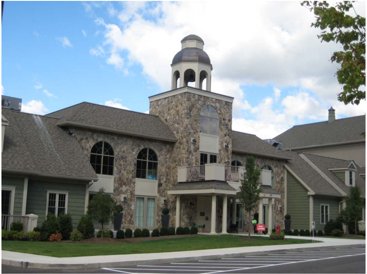
River Village is a new 3 story, 56 unit condominium development that overlooks the Canton River.
